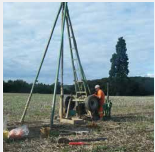
Shell and Auger Drilling
