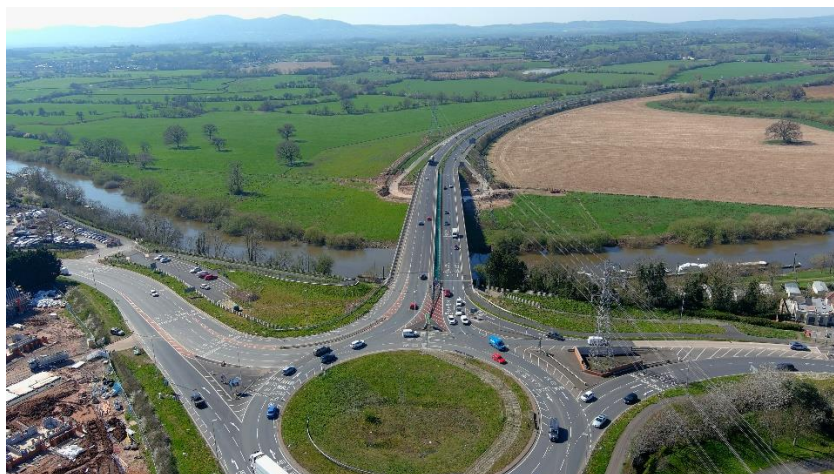
Southern Link Road Phase 4 (SLR4)
