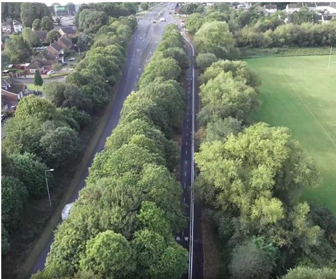
* An ariel view of scheme 2a segregated pedestrian / cycle route parallel to A38.
