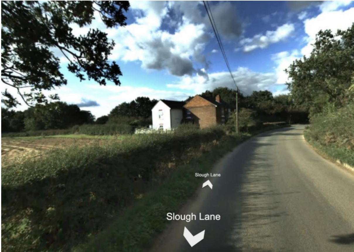
No. 2 Coronation Cottages – Slough Lane. Southern elevation with ground and first floor windows facing soil bund. The toe and crest of screen bund will be 12m and 27m respectively from this property. (Streetview - Bing Maps)
