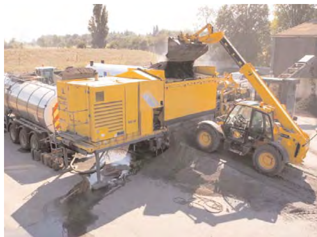
Photo: Stanford Highway Depot processes highway maintenance waste (including tarmac from roads and footways, concrete kerbs and road planings) to produce Type 1 sub-base, storage grade foambas (tarmac) and structural grade foambase. All Type 1 sub-base used for road maintenance in Worcestershire now comes from this facility rather than from a quarry.
