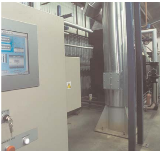
Energy from Waste. Photo courtesy of Recycle Now Partners
