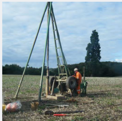
Shell and Auger Drilling
