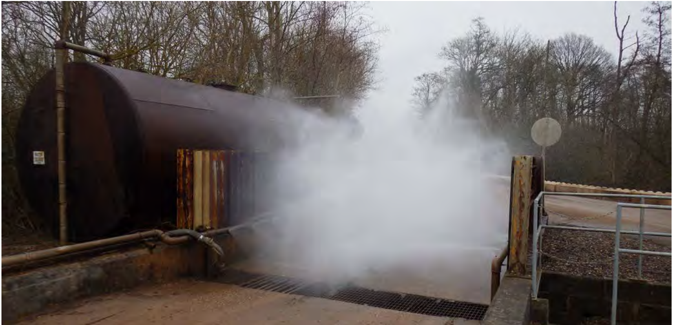
Wheel washing facility at Clifton Quarry
