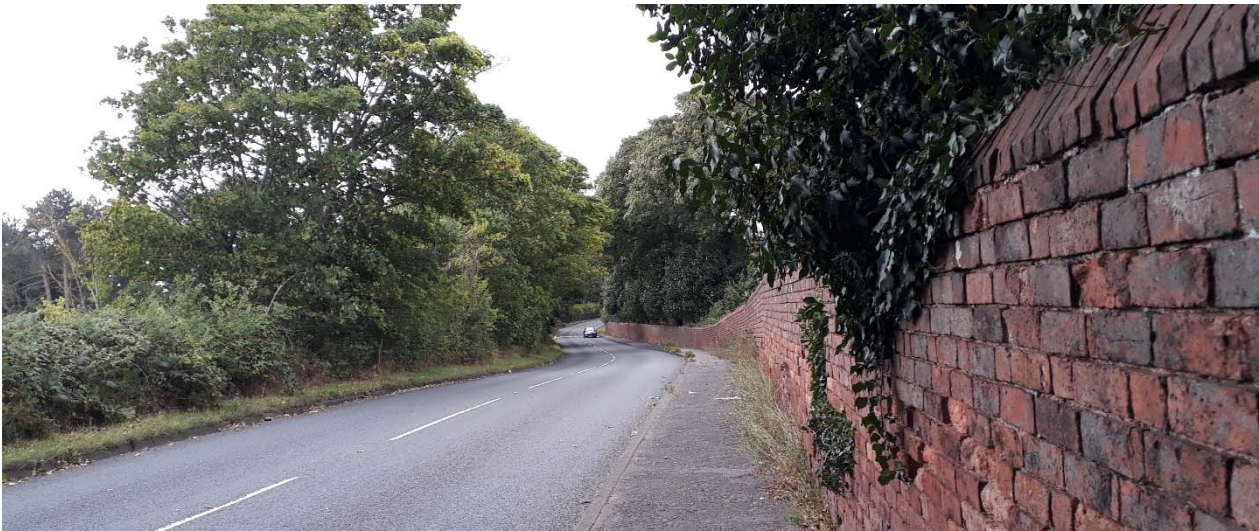
B4189 Wolverley Road looking west towards Sion Hill, showing existing brick wall
