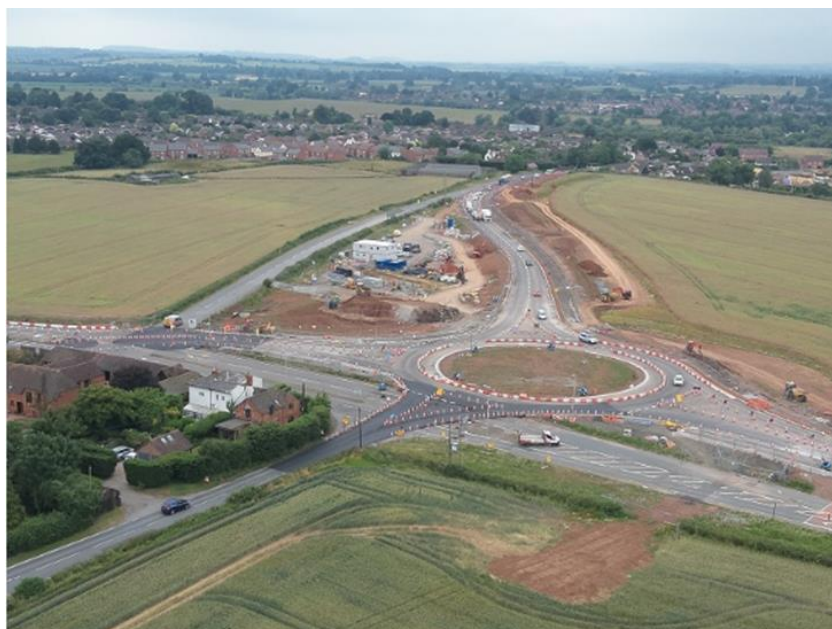
Figure 2: Upton on Severn Junction Improvements
