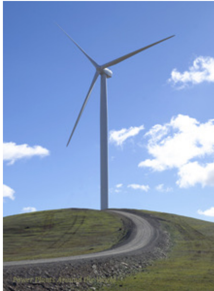
Figure 4 Horizontal Axis Wind Turbine (2.1 MW)
