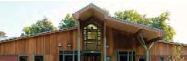
The Cover picture: Redhill Primary School, completed in June 2007, was designed and constructed following an assessment of the impacts of climate change on the new school.
