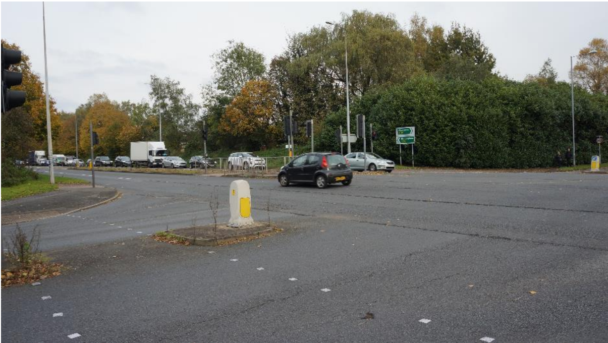
Figure 0.40 – New Road Signals – A38 Crossing provision on route between station and town centre
