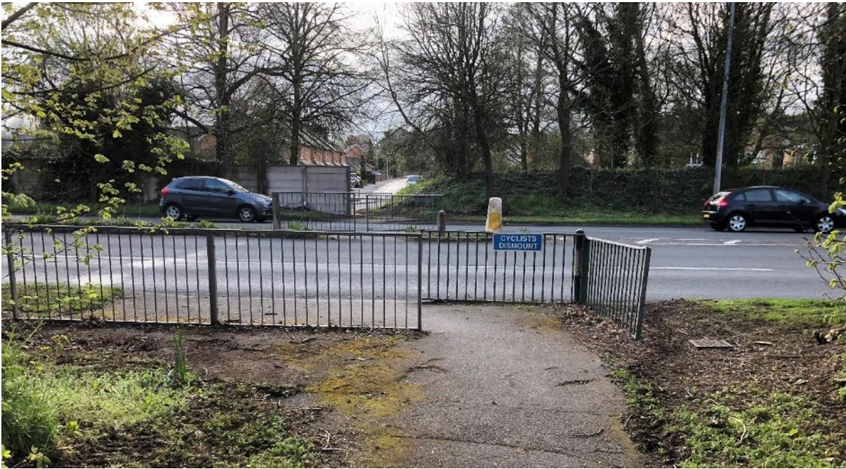
Figure 0.38 - Existing crossing location south of New Road junction
