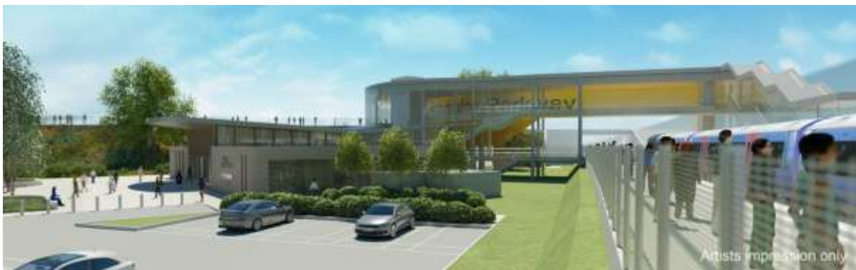
External view of platforms and entrance adjacent to the Birmingham to Bristol Line
