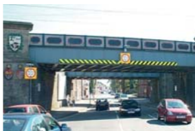
Warning chevrons and circular signs at girder bridge
