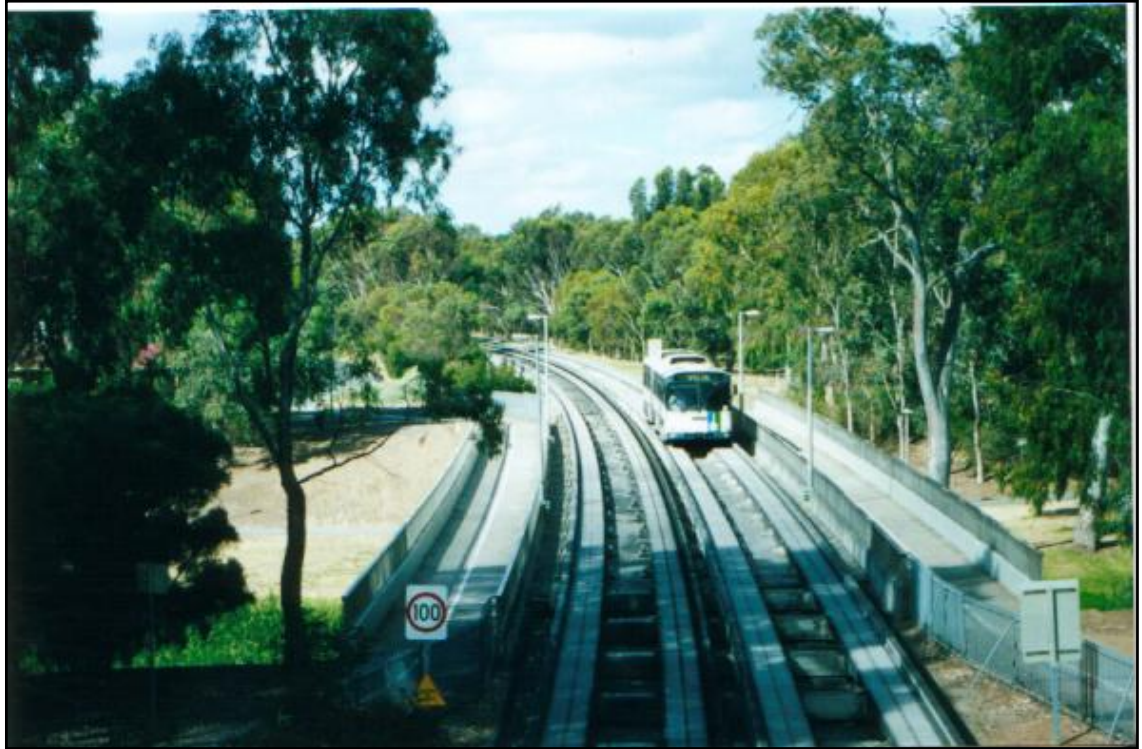
Figure 3.7 - The Adelaide O-Bahn passes along the Torrens Valley.
