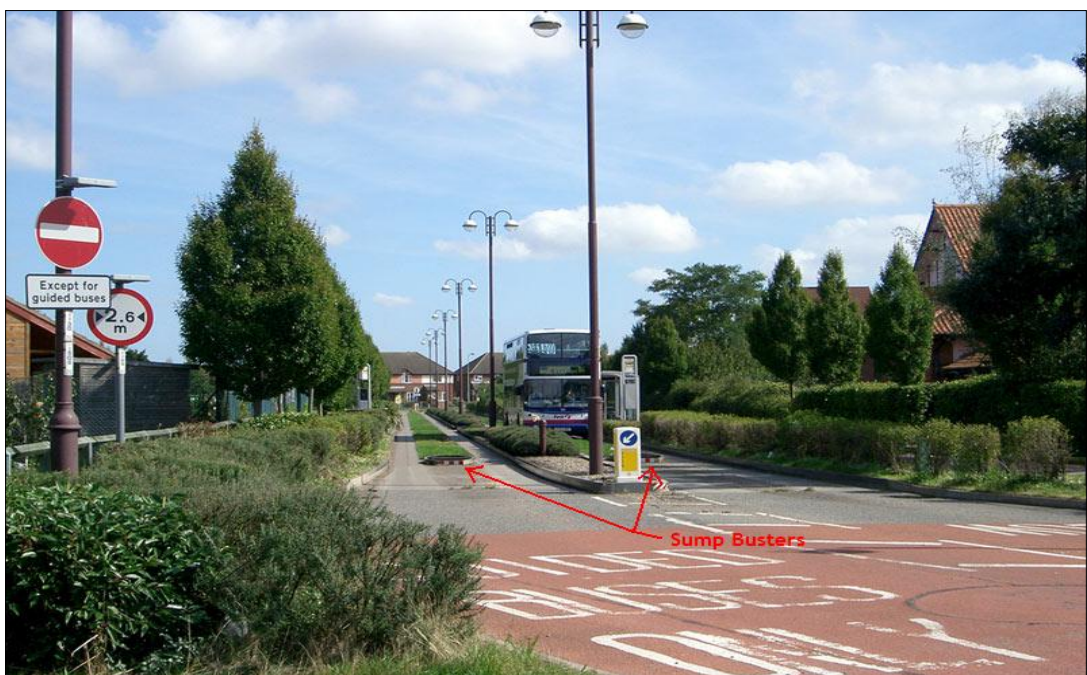
Figure 4.4 - A Sump Buster Installed on a Busway in Ipswich
