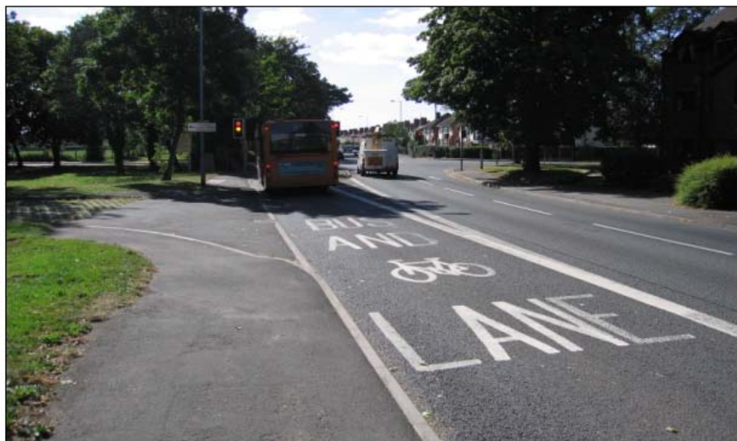
Figure 4.3 - Bus Using a Traffic Signal Controlled Bus Gate on Droitwich Road, Worcester
