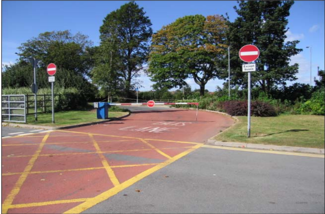
Figure 7.2 - Rising Arm Barrier on Busway at Worcester Perdiswell Park and Ride Site
