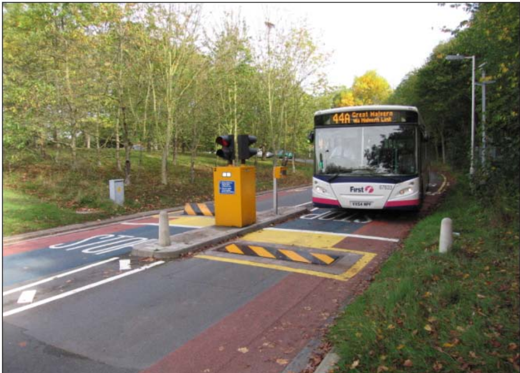
Figure 7.3 - Rising Step Barrier at Worcestershire County Hall, Worcester
