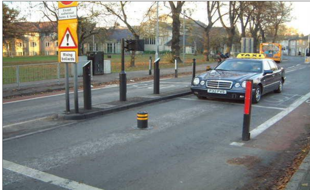
Figure 4.2 - Taxi Using Bus Gate With Rising Bollard in Cambridge
