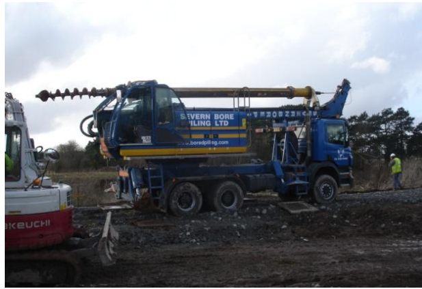
The piling rig moving between locations
