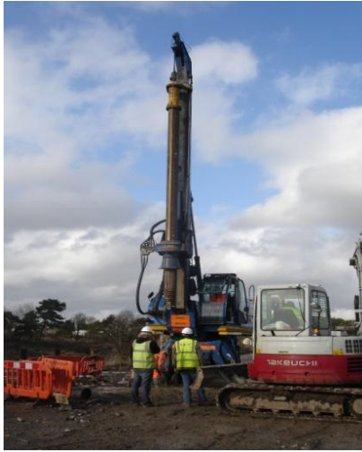
The piling rig at work
