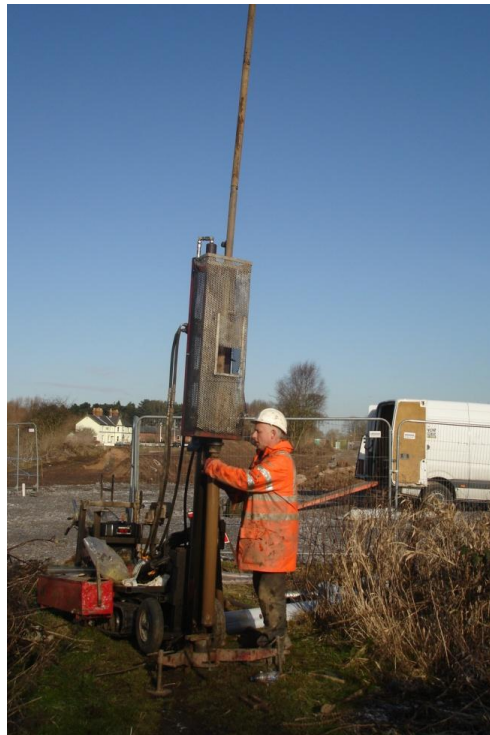
The Archaeological borehole being sunk on the east bank
