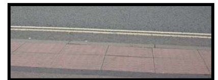
Red Tactile Paving at a Pelican Crossing in Worcester
