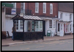
Kassel Kerbing in front of shelter at bus stop in Tenbury
