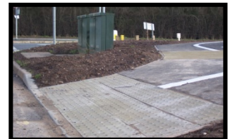
Buff Tactile Paving at A442, Hampton Lovett
