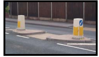
Pedestrian Refuge at Bromwich Road, Worcester
