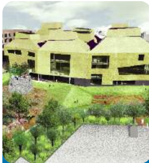
Work continued through 2010-11 on The Hive, which is due to open in 2012 and is set to be Europe's first joint public and academic library, creating jobs for local people.
