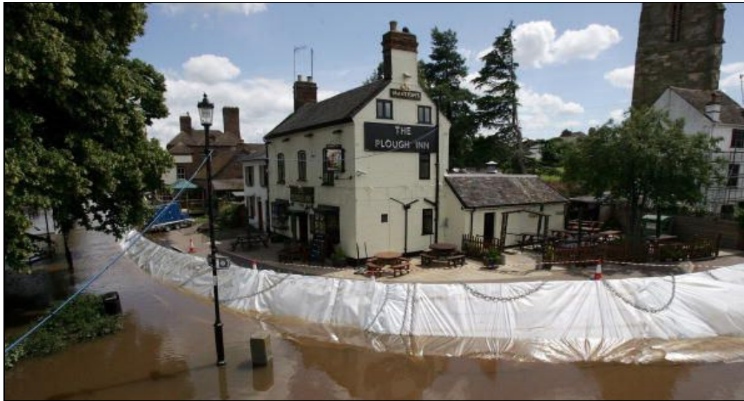
The Plough Inn showing temporary flood defence March 2007
