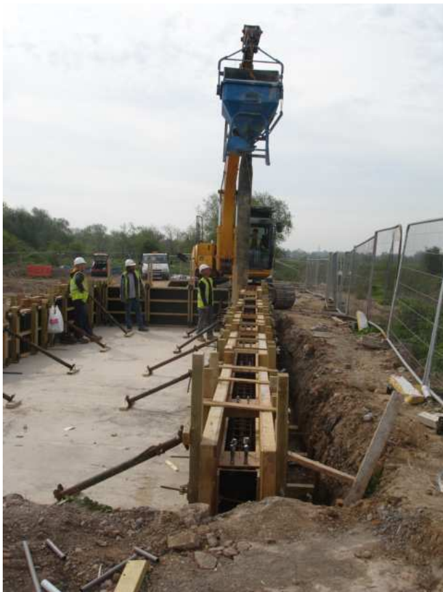
Pouring the concrete into the east bank ramp trough foundation wall
