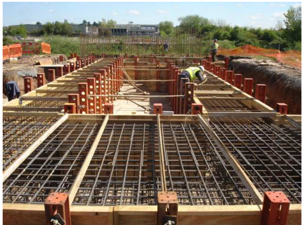
The west bank abutment & anchor block foundation, before concreting
