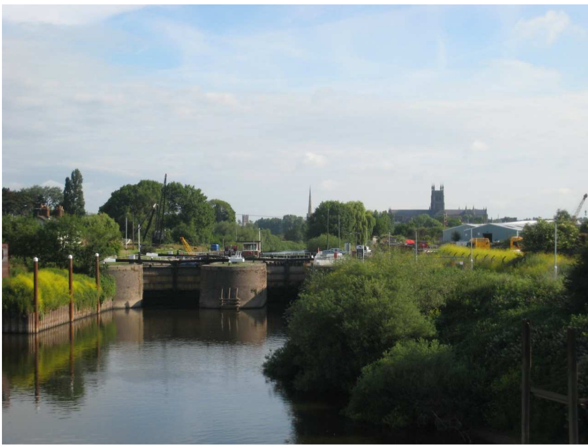
View from the Bridge (North)
