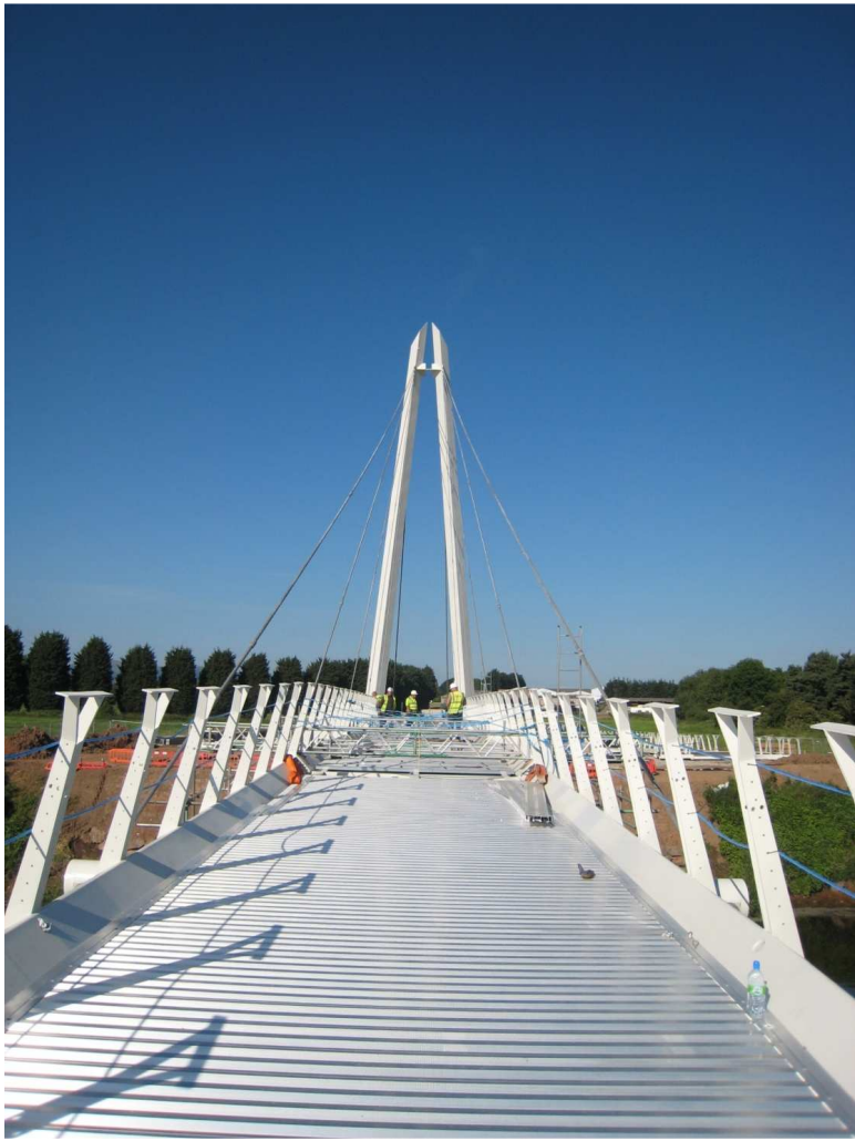
The view on the Bridge from the east bank
