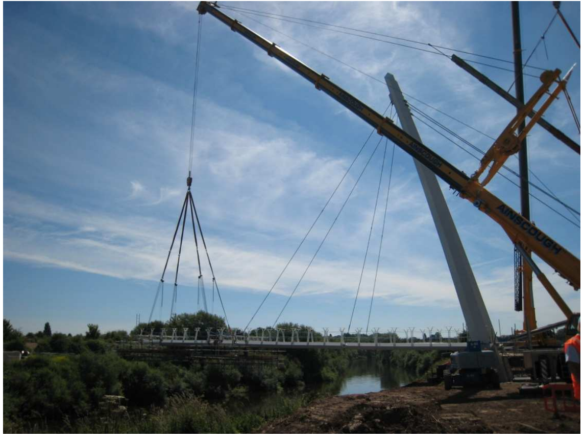
The second 11m long deck section
