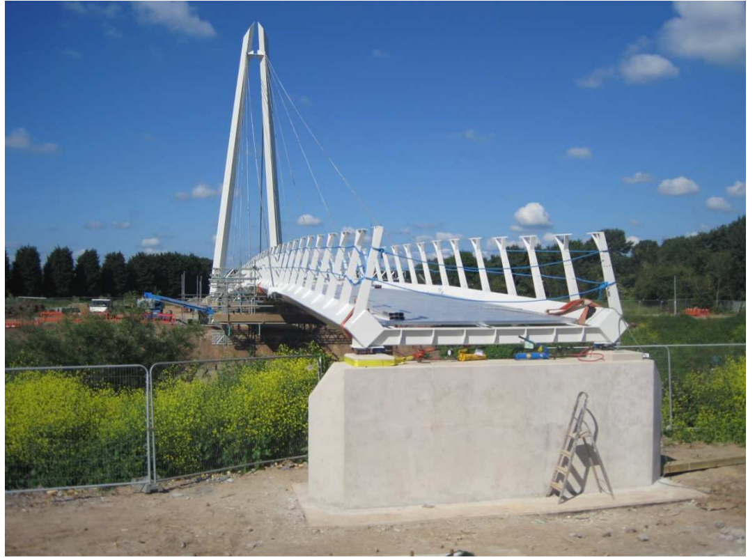
It fits! A tense moment is over for the Project Team.
