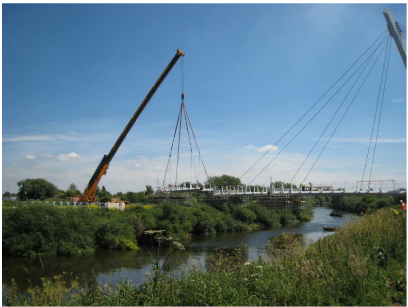
The third 11m long deck section
