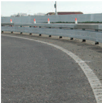
Retro fitted treatment to safety barrier. Highways Agency.
