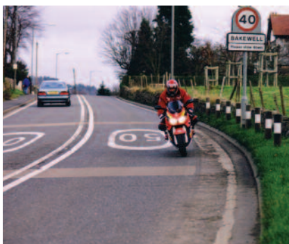
Road markings at the point where motorcycle needs to brake before cornering. Keith Sharples Photography.
