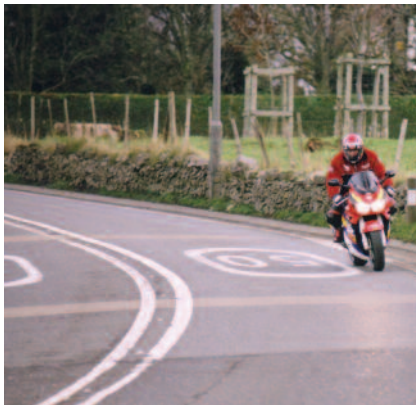
Avoid thermoplastic marking on bends. Keith Sharples Photography.
