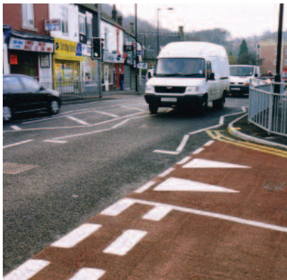
Street furniture can obscure sightline to right, on exit from side road. Keith Sharples Photography.
