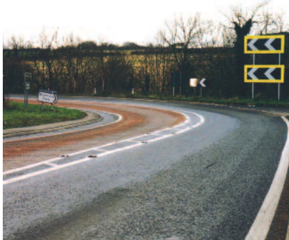
Added warning of hazardous bend. Keith Sharples Photography.
