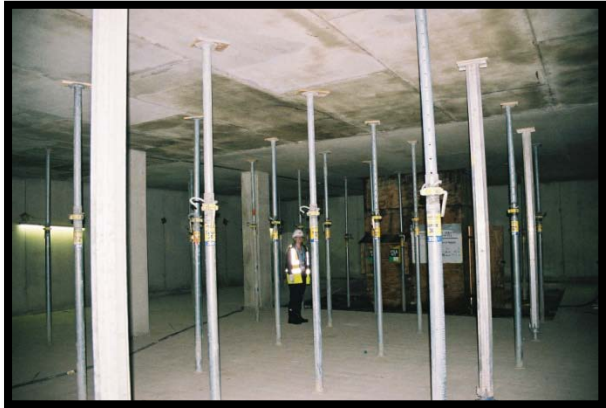
One of the completed archive stores
