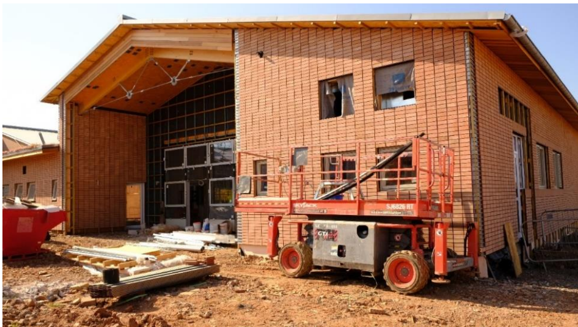
Figure 5: Holyoakes Field First School Construction
