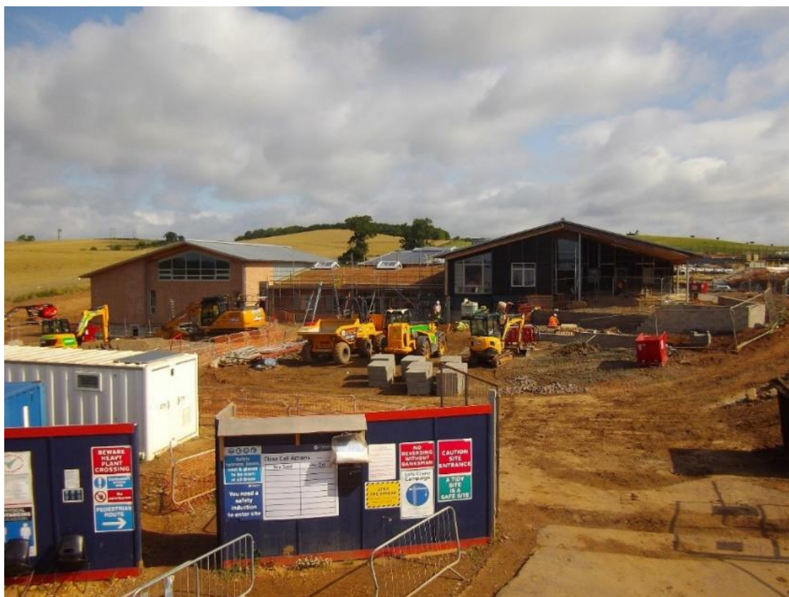
Figure 4: Holyoakes Field First School Construction
