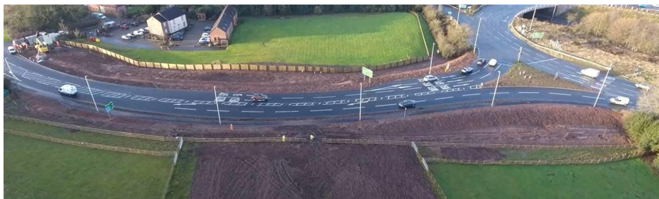
Figure 2 Improvements Completed at M5 Junction 4 (A38)
